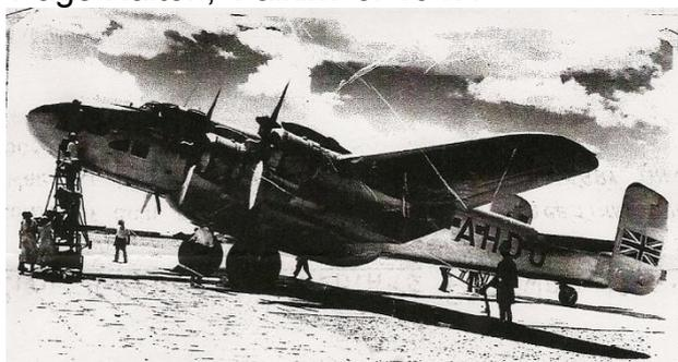
Using the basic 'Halifax' bomber design Handley Page produced the civil Halton as a temporary stopgap. Twelve of these aircraft were ordered by B.O.A.C and used on the London to Karachi service, where the picture above was taken. They first entered service on 1<sup>st</sup> July 1947. They were all withdrawn from B.O.A.C on 2<sup>nd</sup> May 1948 and sold to other users and later operated by Bond Air Services, they played a leading role in the Berlin airlift.
